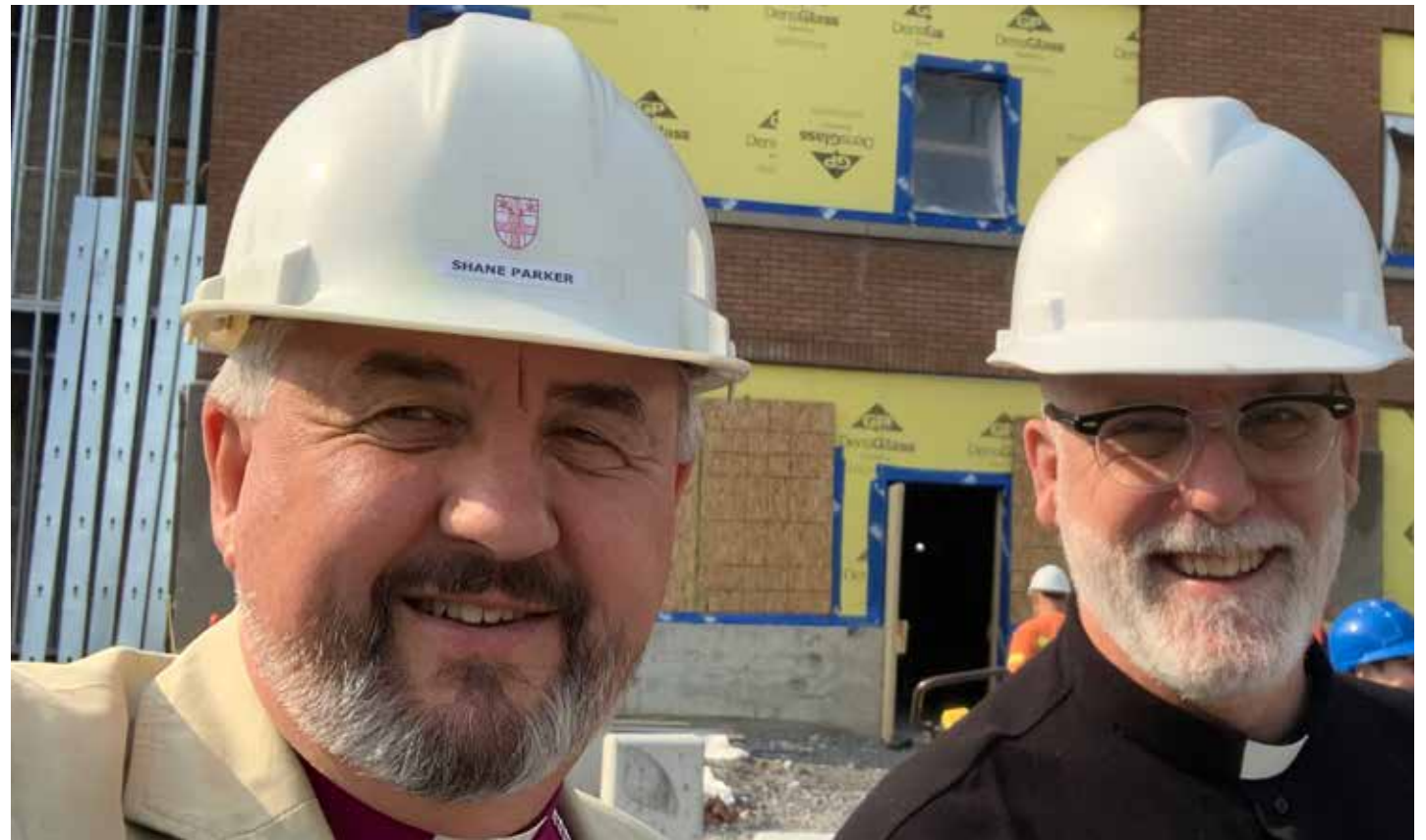
Bishop Shane Parker and the Rev. Canon Peter John Hobbs, director general of the Anglican Community Ministries, on site at Cornerstone Housing for Women's Eccles Street building, formerly an office building that is being renovated to provide supportive housing. PHOTO: CONTRIBUTED
